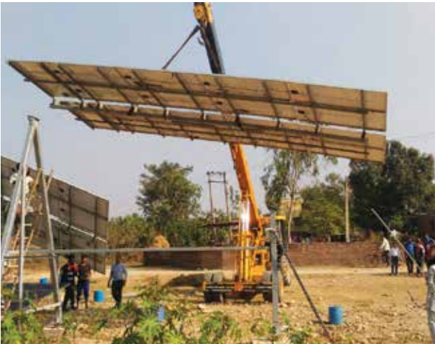
Solar Tracker Installation
