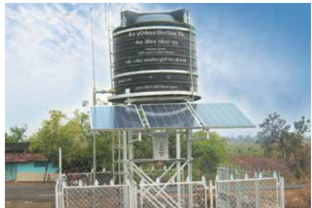
Rural Water Supply Scheme
