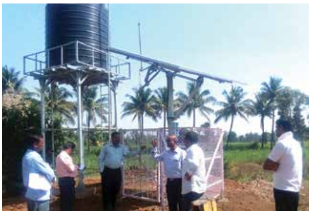
Rural Water Supply Scheme
