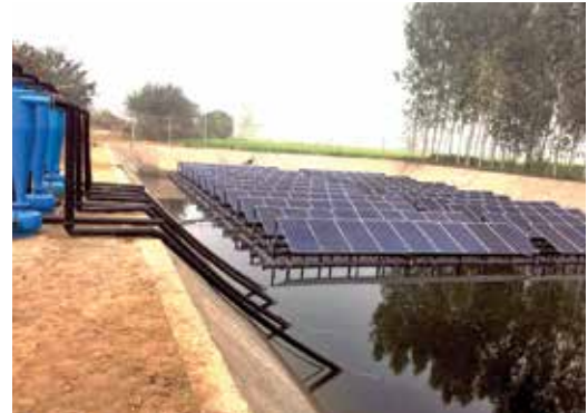
Submersible pump testing
