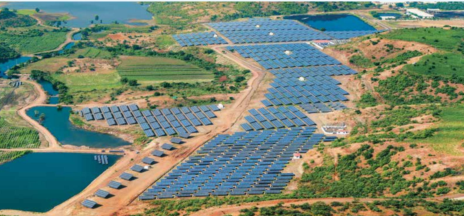
8.5 MWp Solar Power Generation Plant at Jain Valley, Jalgaon
