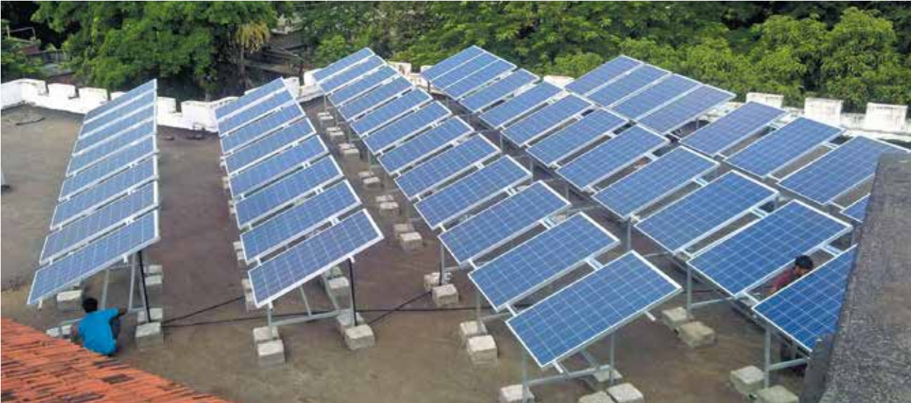
Roof Top Structure
