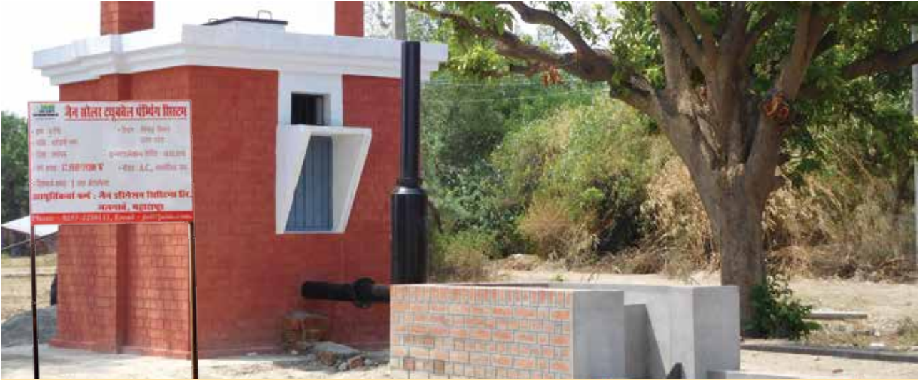
Community Tube Well Pump House
