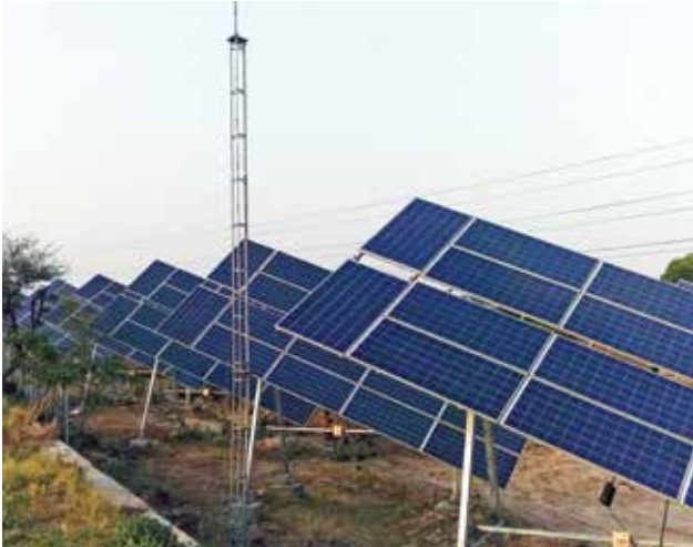
Solar Trackers Installation
